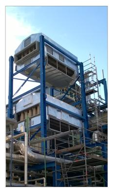
Figure 6 HeatMatrix air preheater in a fired heater
